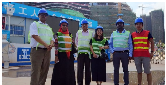
Ethiopian Ministerial Delegation visit to a construction site of Rising Hongfa in Guangxi, China
